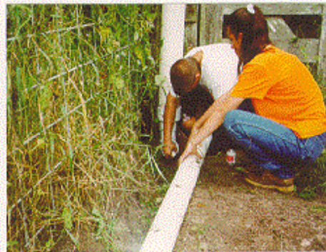
Installation of pipe extension for roof
