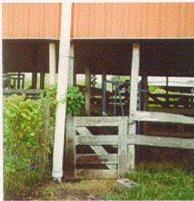
Roof runoff management
