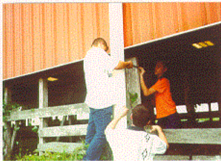
Securing pipe for roof runoff
