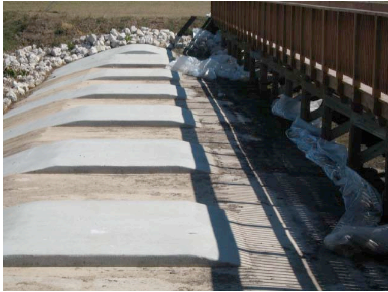
Figure 5 Outfall Weir for Pond
