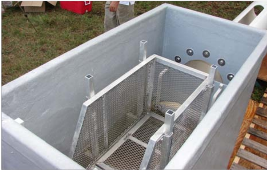
Figure 1 - Sieve strainer screen of Type 2 baffle box
