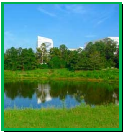
Stormwater pond within the Capital Cascade Greenway and Stormwater Treatment Project
