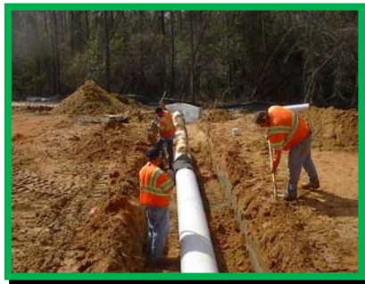
Men install stormwater lines under a soon-to-be-paved road.
