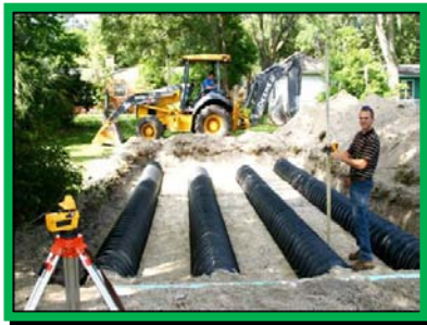
A DOH staffer inspects a drainfield.
