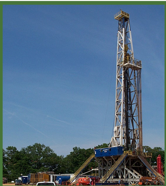
Horizontal well drilling at Jay Field
