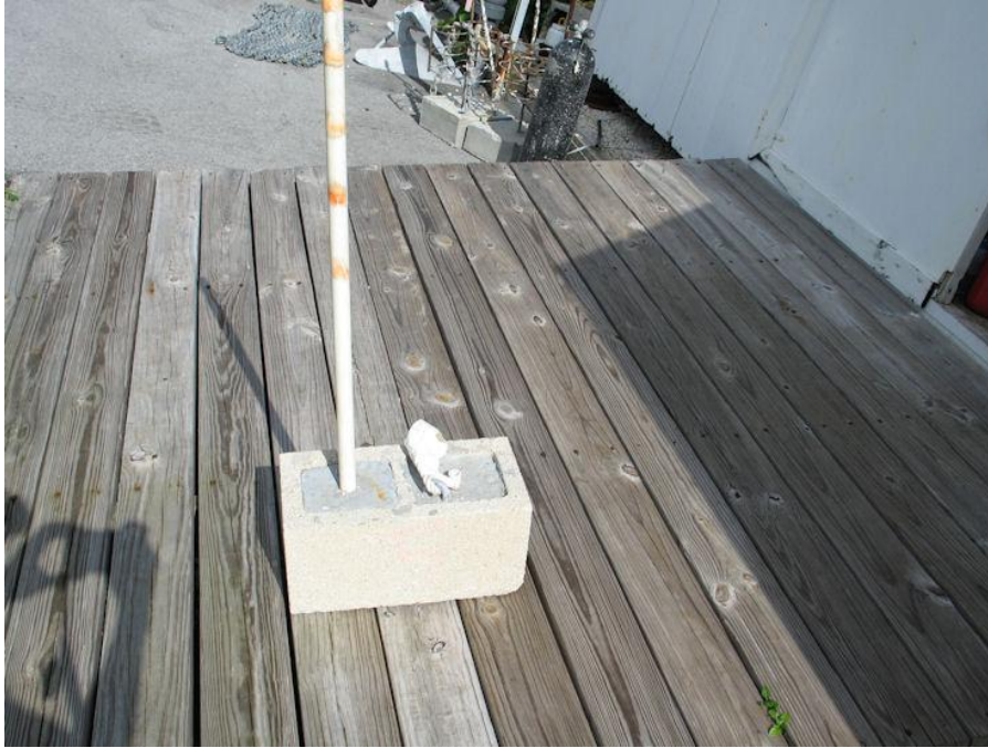
Figure 1. One of 20 concrete-filled cinder blocks used to create a grid in the tire field. This grid was used to by divers to know their locations during the removal operation and late to aid in productivity determination.
