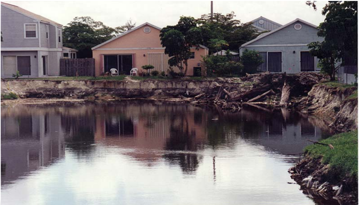
Figure 2 – Hampshire Homes Subdivision Waste Excavation Area
