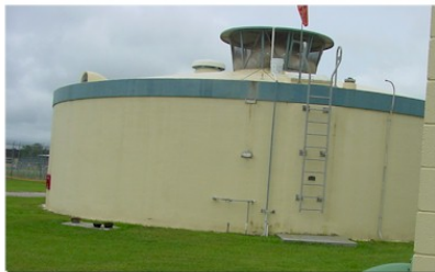
A view of a Wastewater Treatment Plant from the outside
