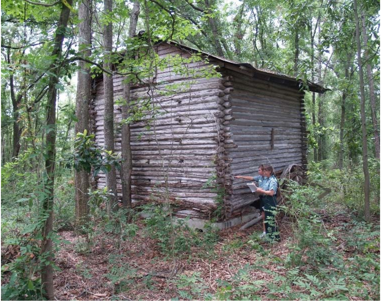
Park staff evaluating a state park historic structure.
