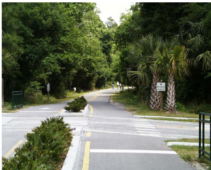
Figure 3. Raised Median Intersection (Courtesy of Seminole County)
