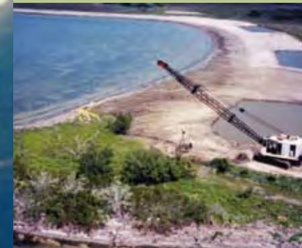
Volusia County restoring wetlands to historic elevations by removing spoil material
