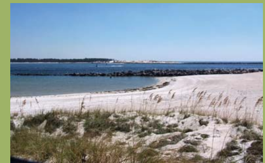
Rock jetties to protect the beach
