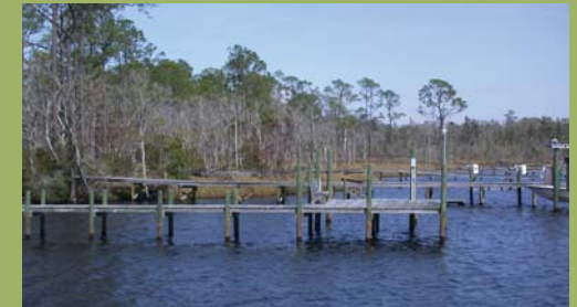
Residential docks along Rocky Bayou preserve
