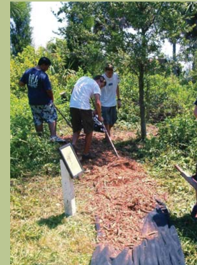
Building an interpretive trail as part of an Eagle Scout project
