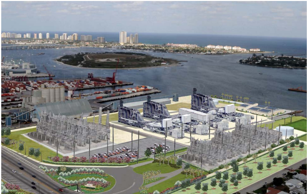
This new power plant, called Riviera Beach Next Generation Clean Energy Center, a $1.3 billion state-of-the-art combined-cycle natural gas plant, will use 33% less fuel for the same production as the previous one, and will sharply reduce greenhouse gas emission and air pollution
