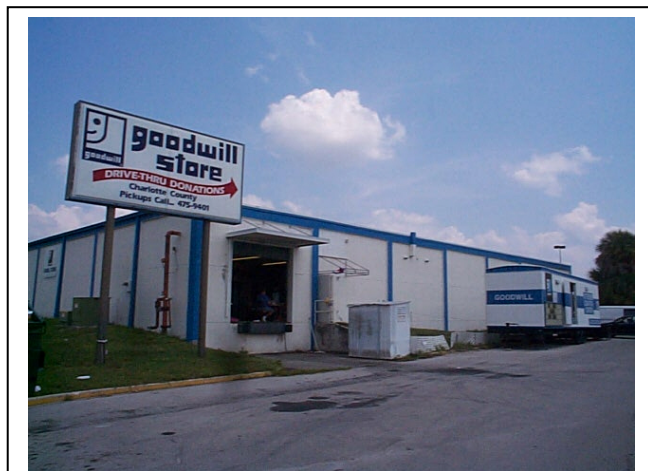
The side view of the Goodwill retail store located in Englewood, FL (Charlotte County). The Electronics Specialty Retail Area and Reuse/Recycling Processing area was located in this facility.
