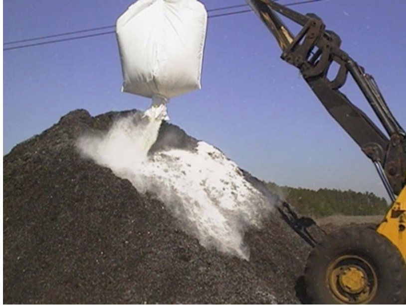
Ground polystyrene being added to compost pile.
