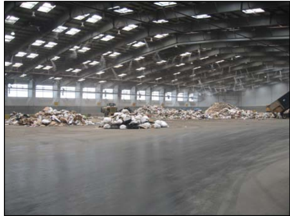
Figure 3.24: Puente Hills Transfer Station with Skylights
