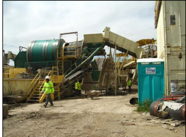
Figure 3.13: Demolition Debris Recovery Line at Zanker Road
