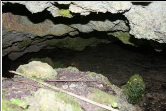
Fissure: a horizontal (sideways) crack in limestone with a measurable length and depth; water may be present inside.
