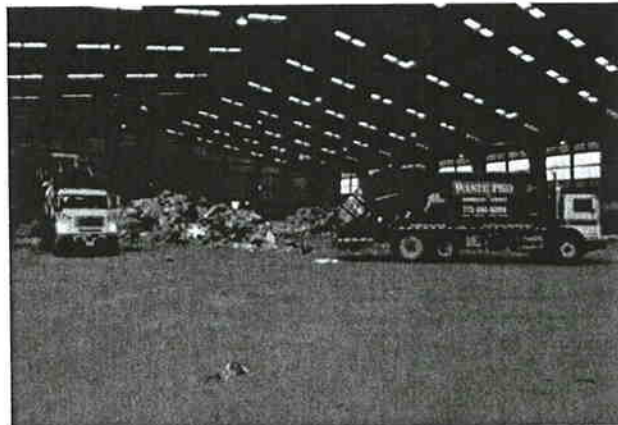
Figure 3. Tipping Floor of Baling and Recycling Facility
