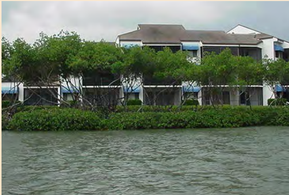
Windowed Red Mangroves along a residential complex
