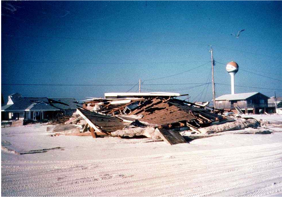
Figure 57. Escambia County - Example of destroyed major habitable structure in Pensacola Beach.
