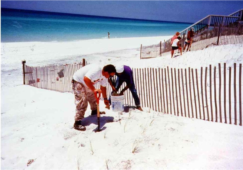
Figure 67. Dune restoration work; sea oat planting and sand fencing; Panhandle Coast.
