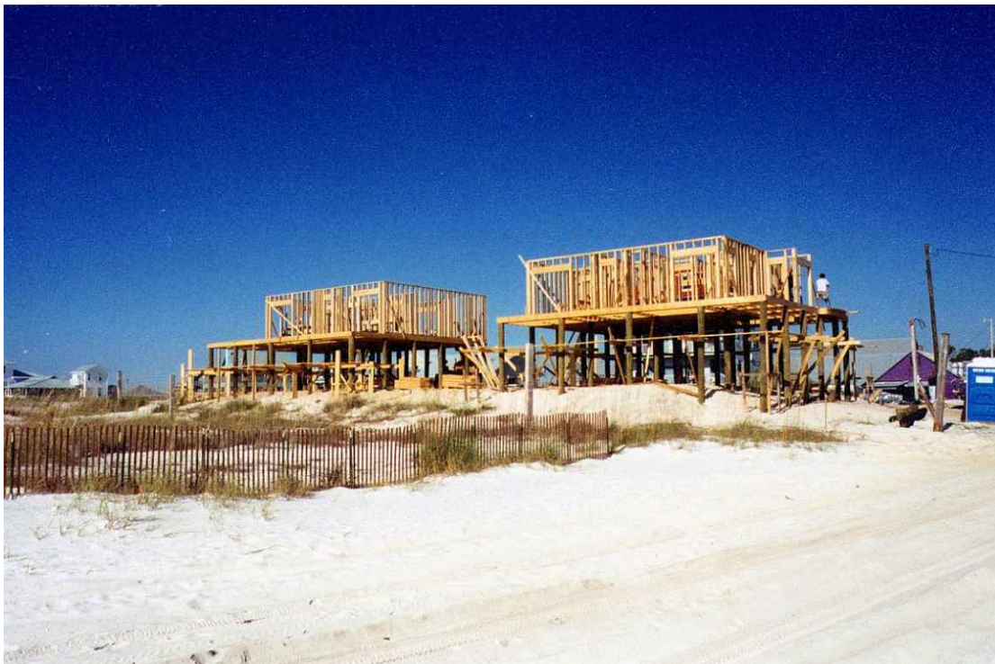
Figure 81. FDEP-permitted habitable structures under construction following Opal.
