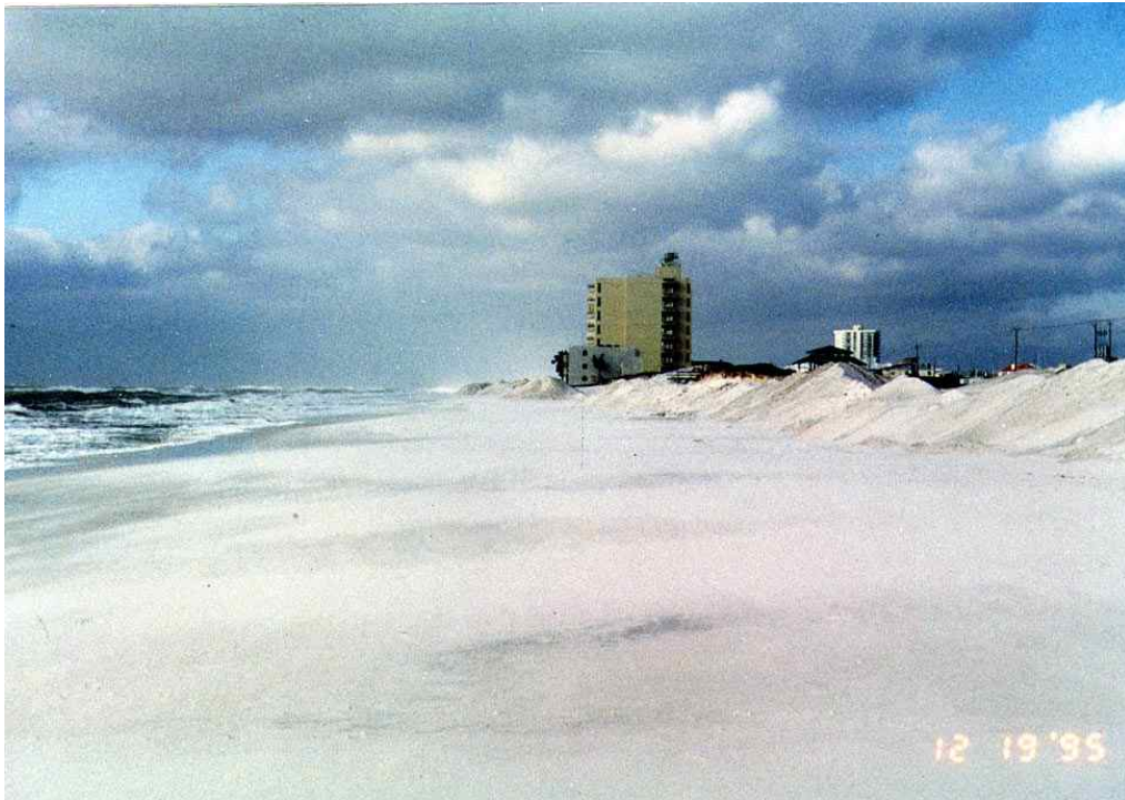
Figure 78. Redistributed sand recovered from overwash following Opal which was trucked back to eroded dune areas in the Pensacola Beach area.
