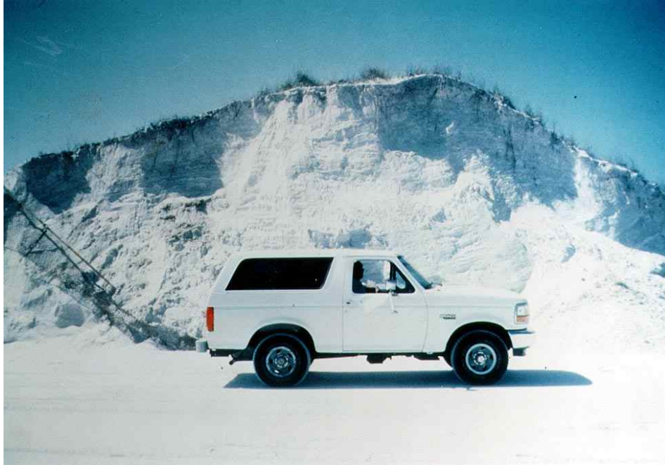
Figure 55. Severe dune breach resulting from overwash in Escambia County (Direction of overwash is from left to right; ie, Gulf of Mexico to left, inland to right).
