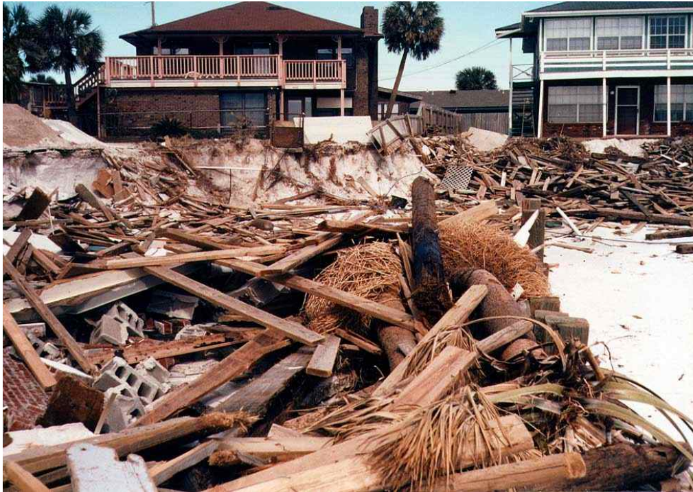
Figure 64. Typical Storm Debris in Panhandle Areas Following Hurricane Opal (Spyglass Drive area of Panama City Beach)
