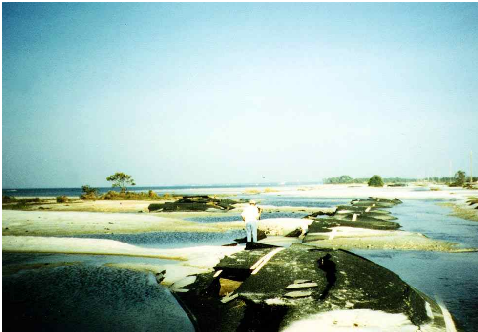
Figure 52. Ground-level photo of the washout of U.S. Highway 98 just east of Ft. Walton Beach resulting from Hurricane Opal overwash (bay to left, Gulf to right).
