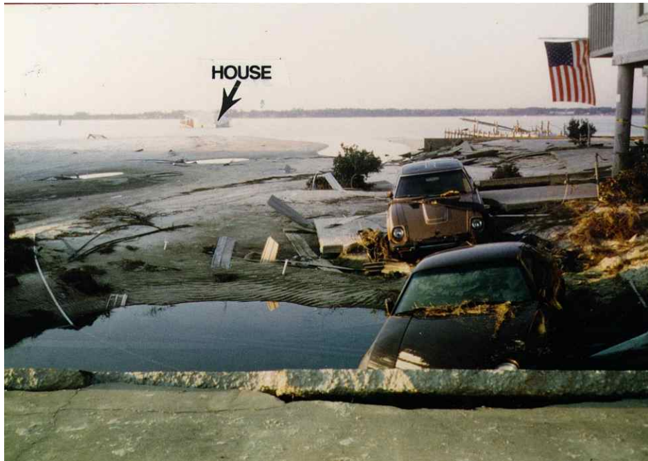
Figure 51. Overwash deposition near Navarre Beach, Santa Rosa County. Note house transported by Opal and deposited into Santa Rosa Sound in the background.
