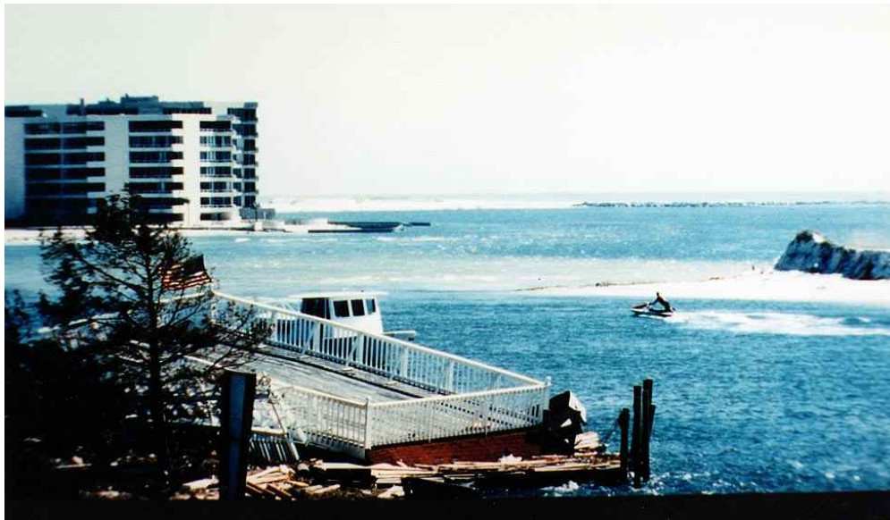
Figure 54. Ground-level view of breach through Norreigo Pt. At Destin-East Pass (looking toward Gulf of Mexico from Old Pass Lagoon).
