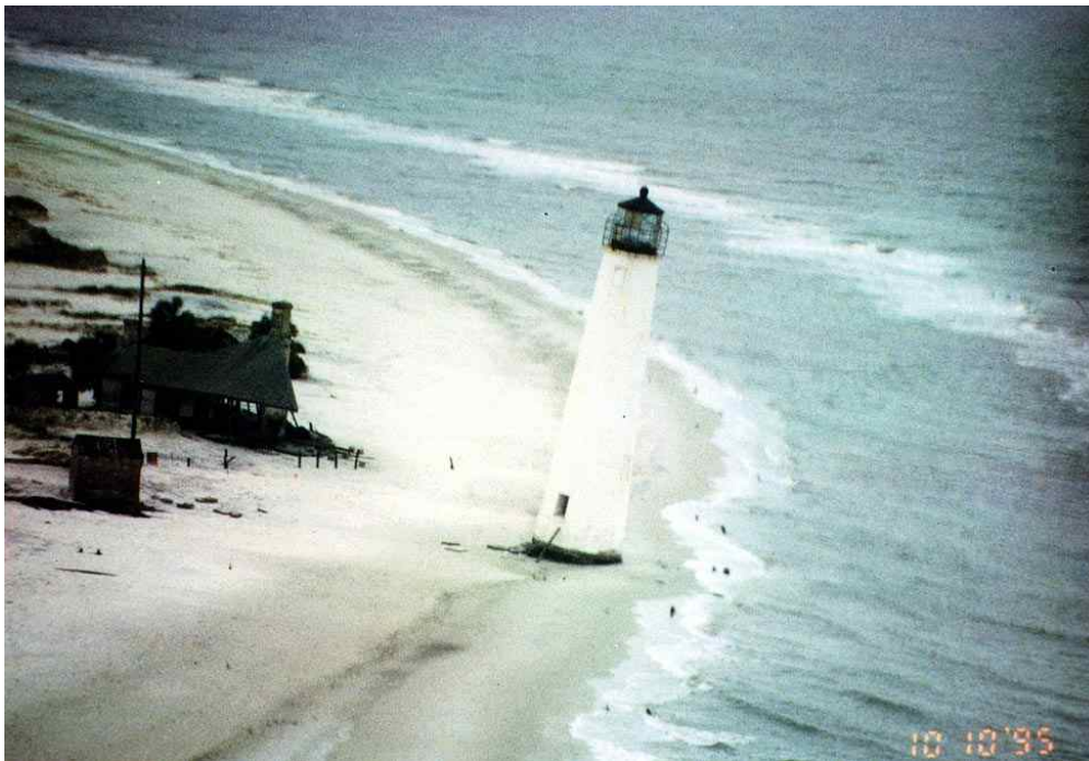
Figure 56. Cape St. George Lighthouse on Little St. George Island (already severe erosion area significantly worsened by Hurricane Opal).
