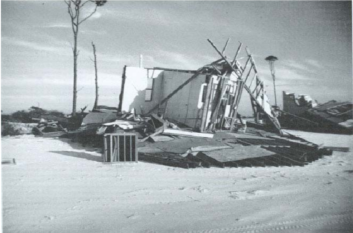
FIGURE 16. Dwelling destroyed, St. Joseph Peninsula.
