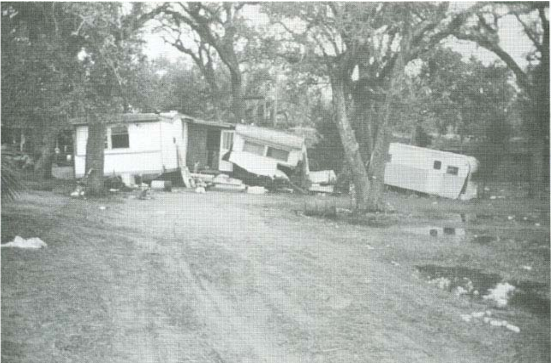
FIGURE 103. Mobile home damaged by flooding, Spring Creek.
