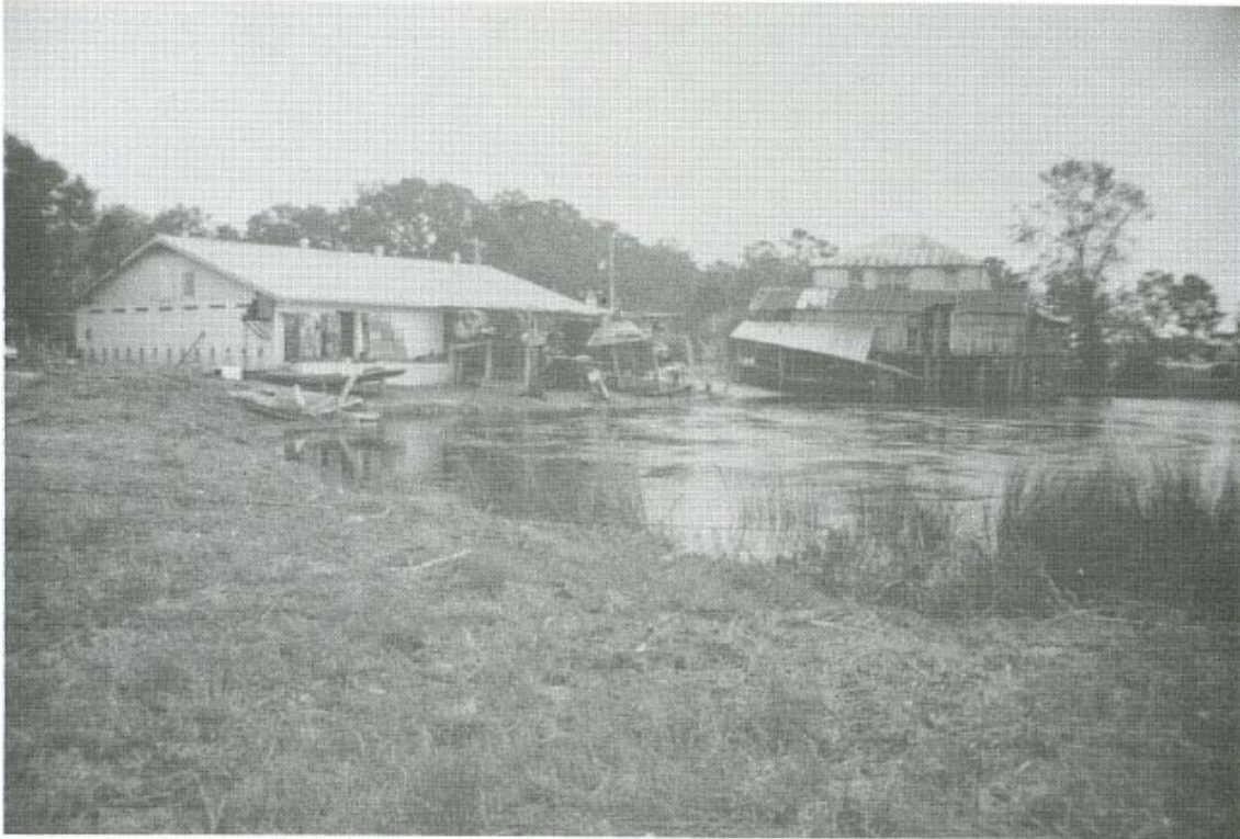
FIGURE 102. Damage to Spring Creek seafood processing plants.
