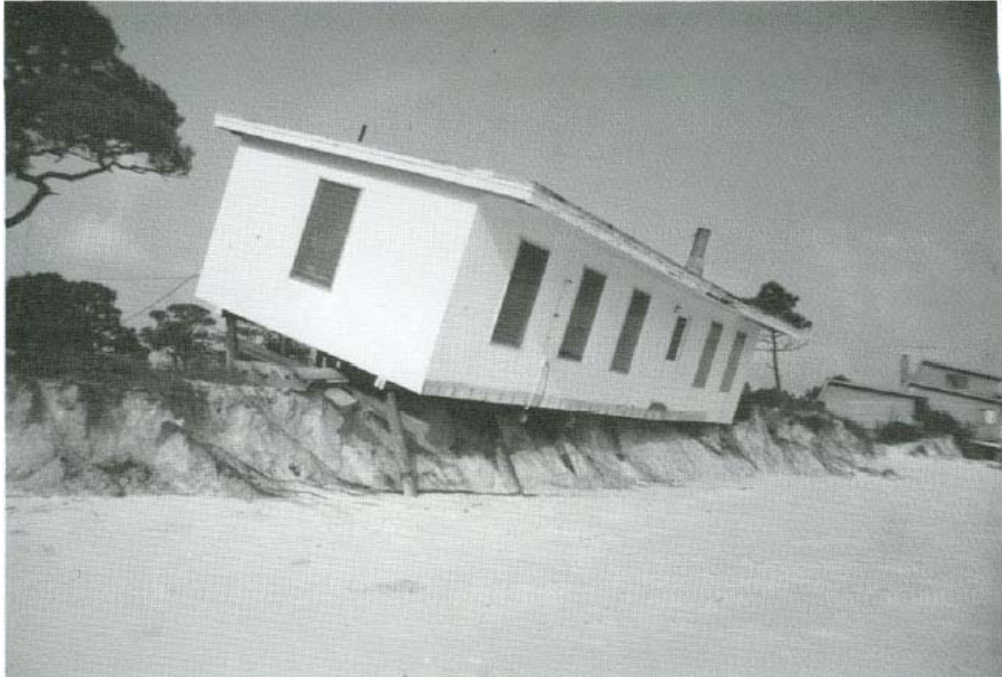
FIGURE 96. Lighthouse Point dwelling damaged by Kate's erosion.
