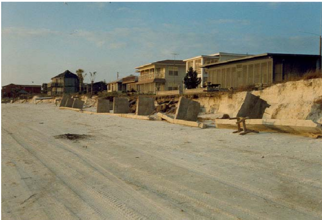
FIGURE 11. Concrete wall destroyed, Mexico Beach (Brett D. Moore).
