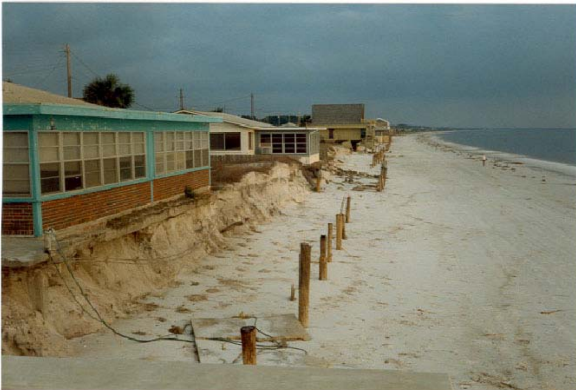
FIGURE 10. Mexico Beach Dwellings Threatened by dune erosion (Brett D. Moore)
