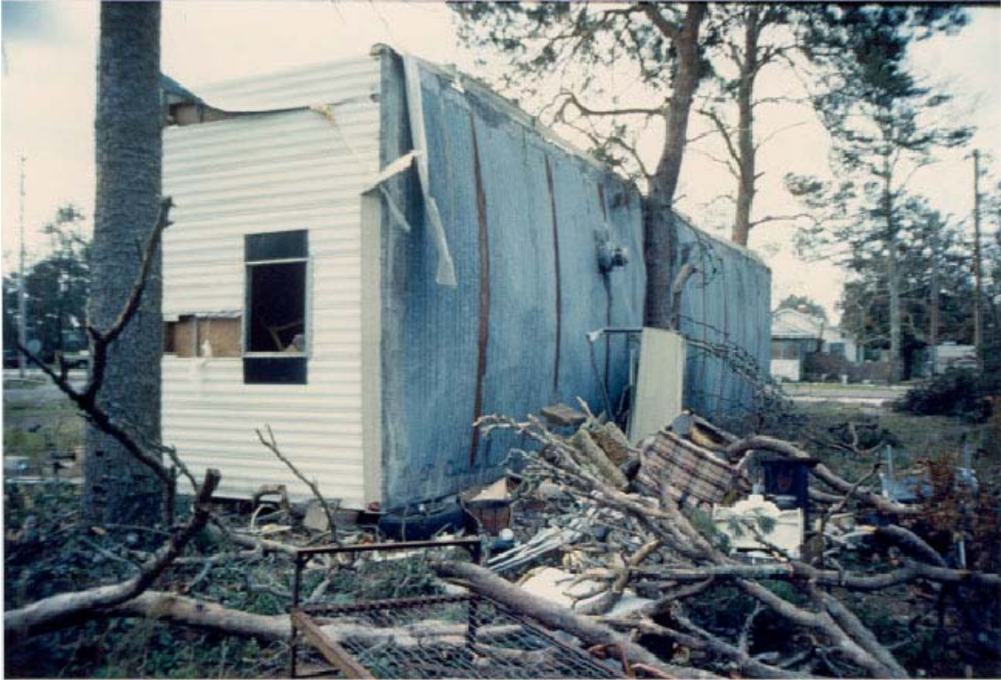
FIGURE 79. Mobile home rolled by downburst behind the Carrabelle IGA Food Store.
