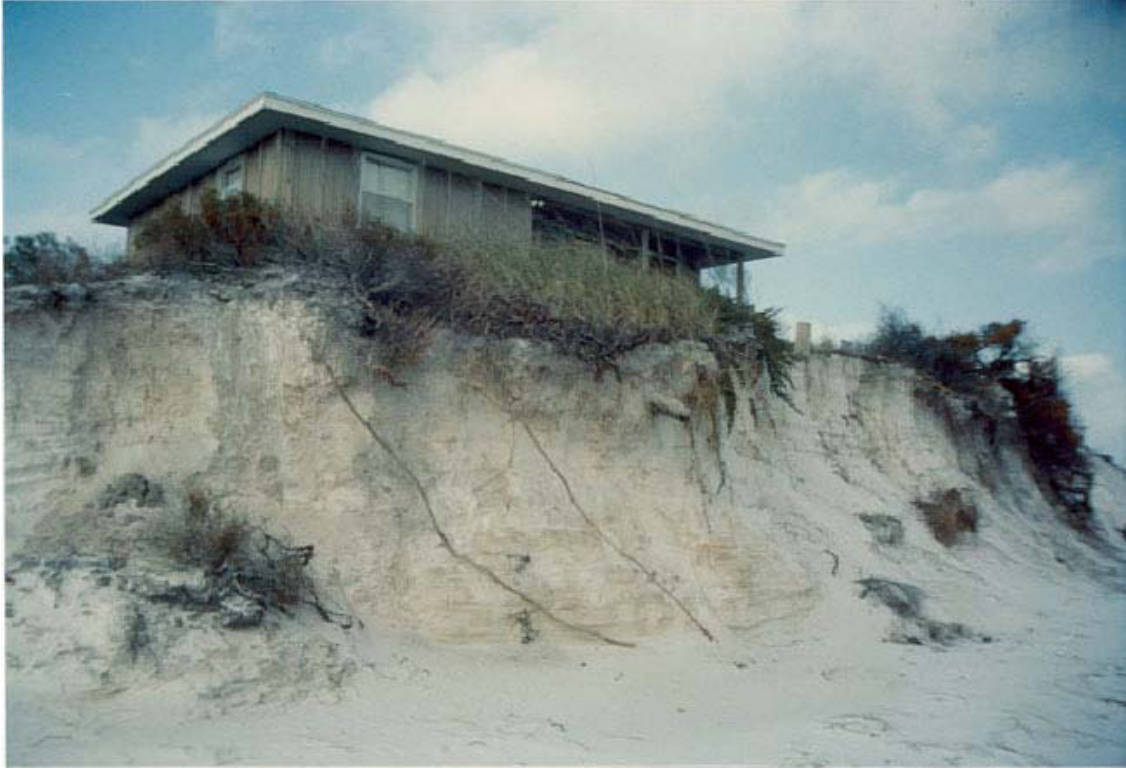
FIGURE 61. Severe erosion threatens dwelling, Dog Island.
