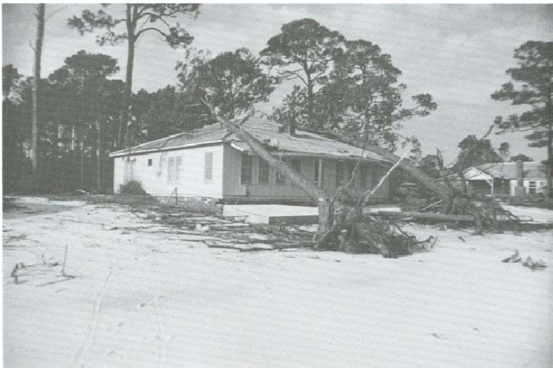
FIGURE 72. Dwelling damaged by two toppled pines.
