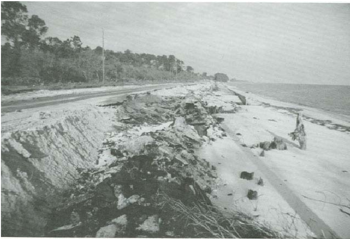
FIGURE 68. U.S. Highway 98 destroyed between Green Point and Yent Bayou.
