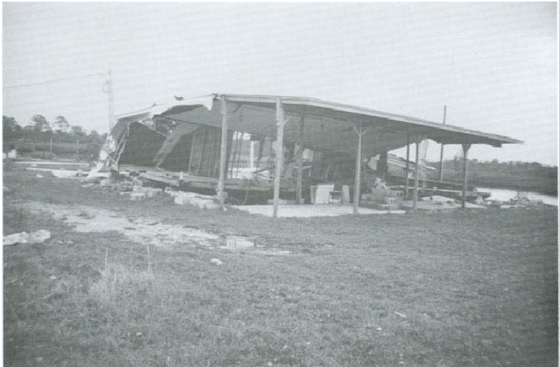
FIGURE 105. Oyster Bay dwelling was destroyed yet screened porch was still standing.
