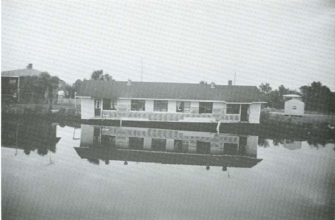
FIGURE 106. Oyster Bay dwelling was carried across the canal by flood waters and deposited on the opposite bank.
