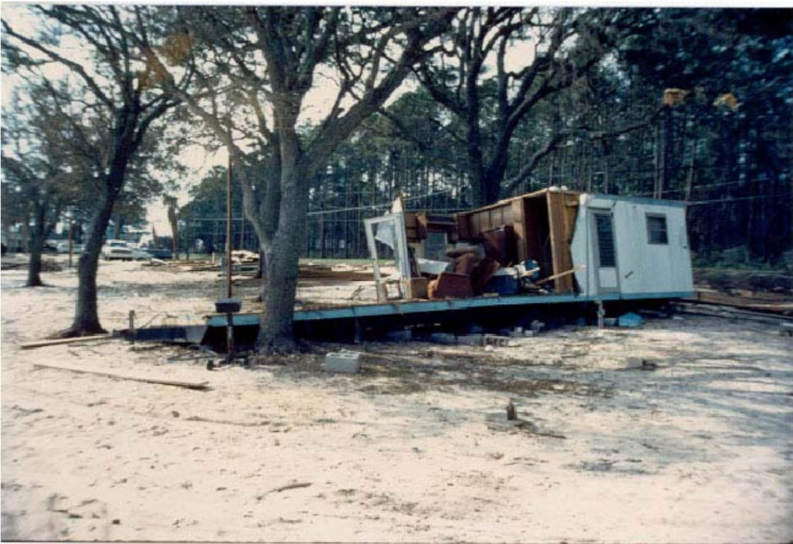
FIGURE 80. Mobile home east of Carrabelle destroyed by battering loads of waterborne debris from house destroyed on Dog Island.
