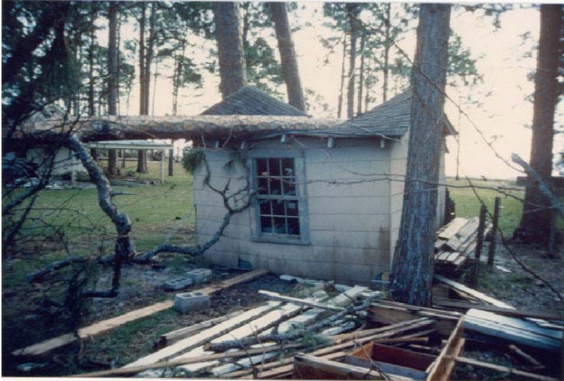
FIGURE 81. One of many fallen pines in St. James.
