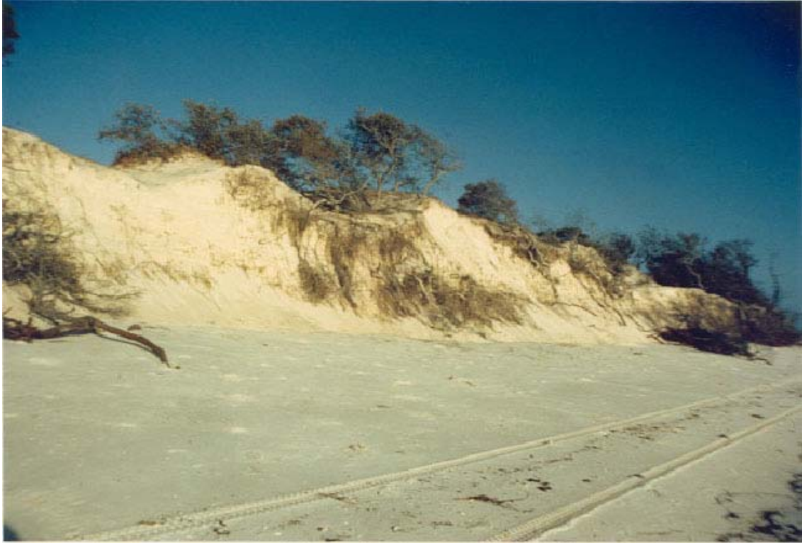
FIGURE 97. Heavy dune erosion between Lighthouse Point and Bald Point.
