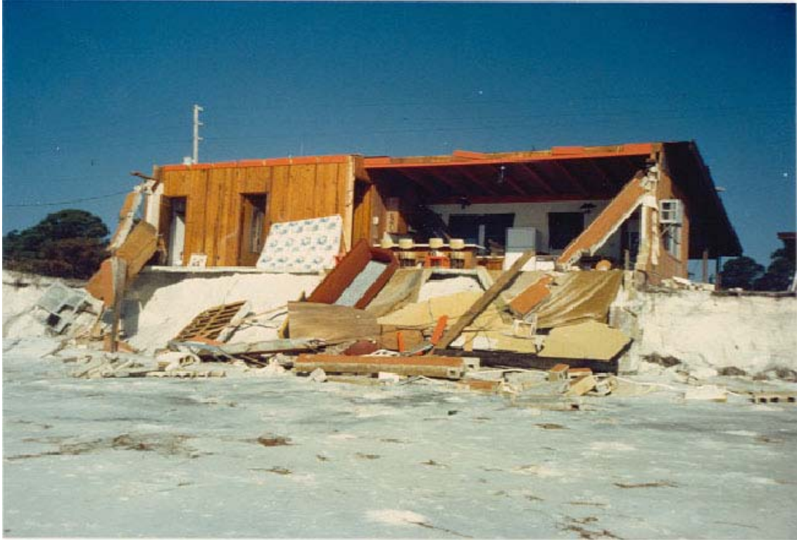
FIGURE 93. Slab-on-grade dwelling undermined and destroyed.
