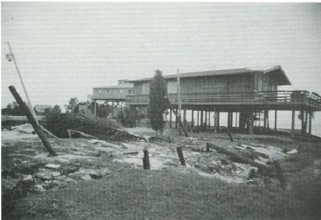
FIGURE 122. Site of the dwelling which was probably hit by a tornado.
