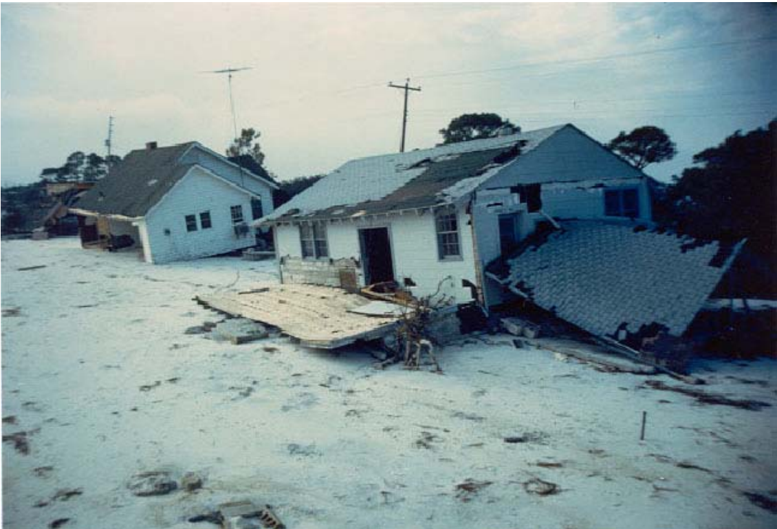
FIGURE 90. Dwellings damage by Elena were additionally damaged by Kate.
