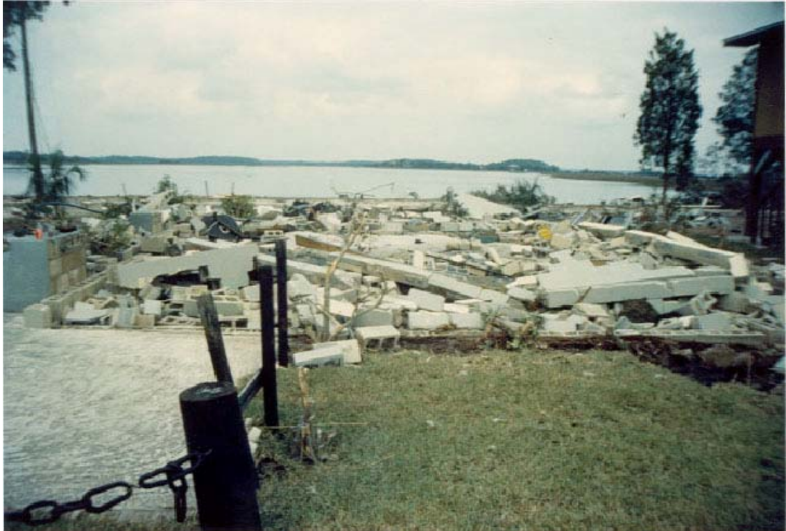
FIGURE 118. Concrete block dwelling pulverized by wave activity.
