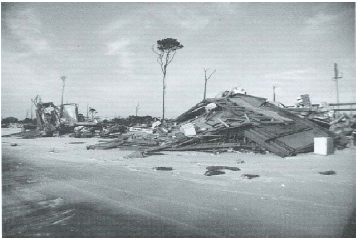
FIGURE 17. Dwelling destroyed, St. Joseph Peninsula.
