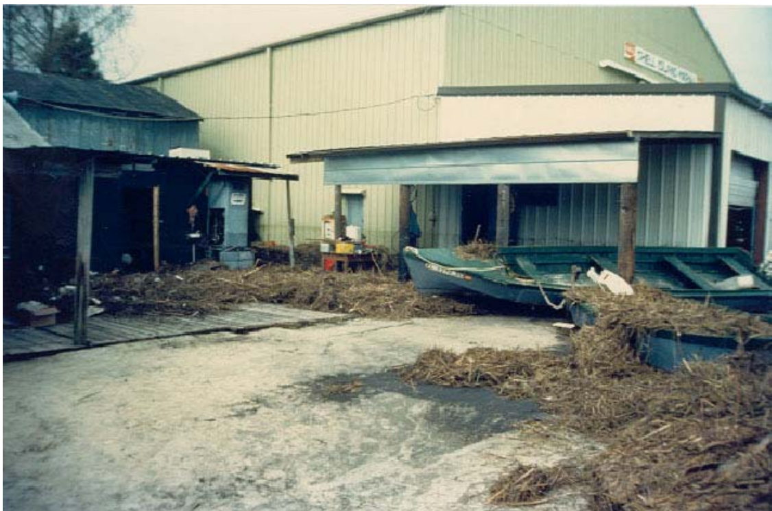
FIGURE 111. Shell Island Marina on the Wakulla River was damaged by flooding.
