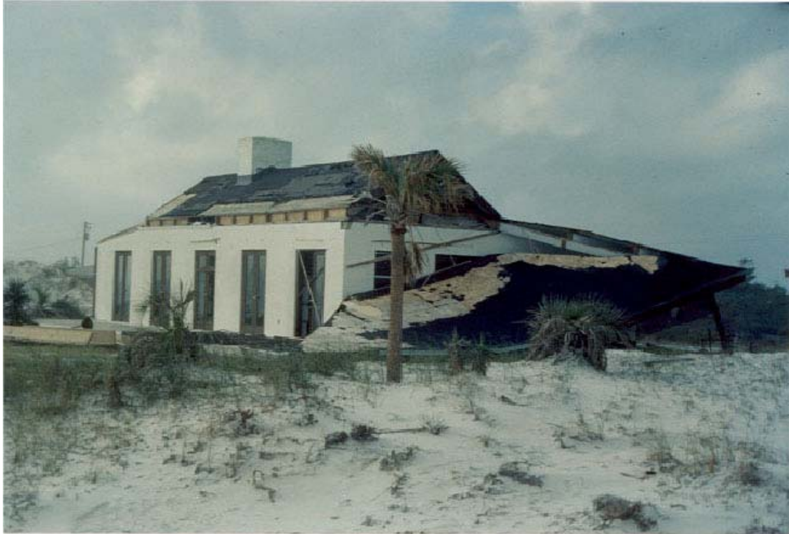
FIGURE 62. Dwelling sustained major structural roof damage due to wind.
