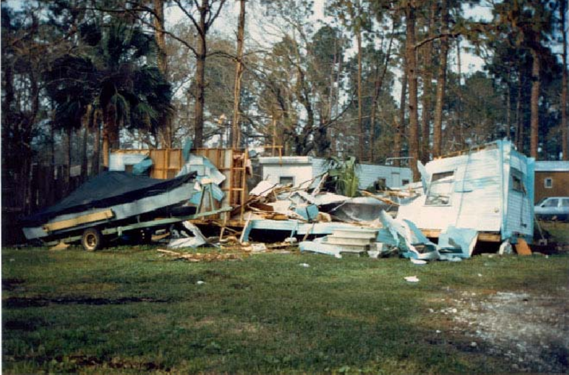
FIGURE 32. Mobile home destroyed by wind.
