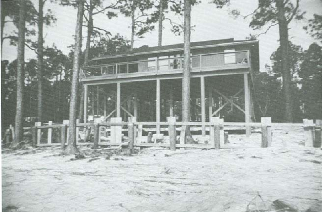
FIGURE 85. Sufficiently elevated dwelling with no damage although wood bulkhead was destroyed.
