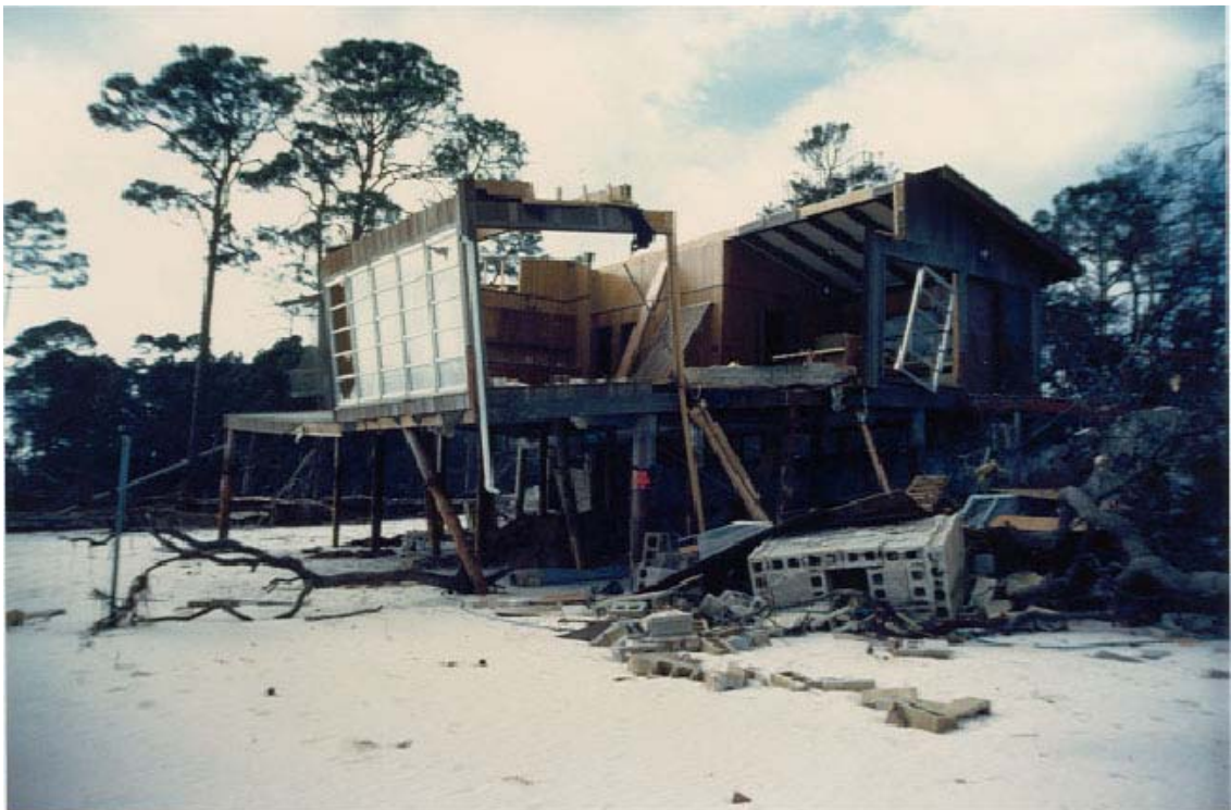
FIGURE 78. Pile-supported dwelling destroyed by wind, waves, and erosion of Kate.
