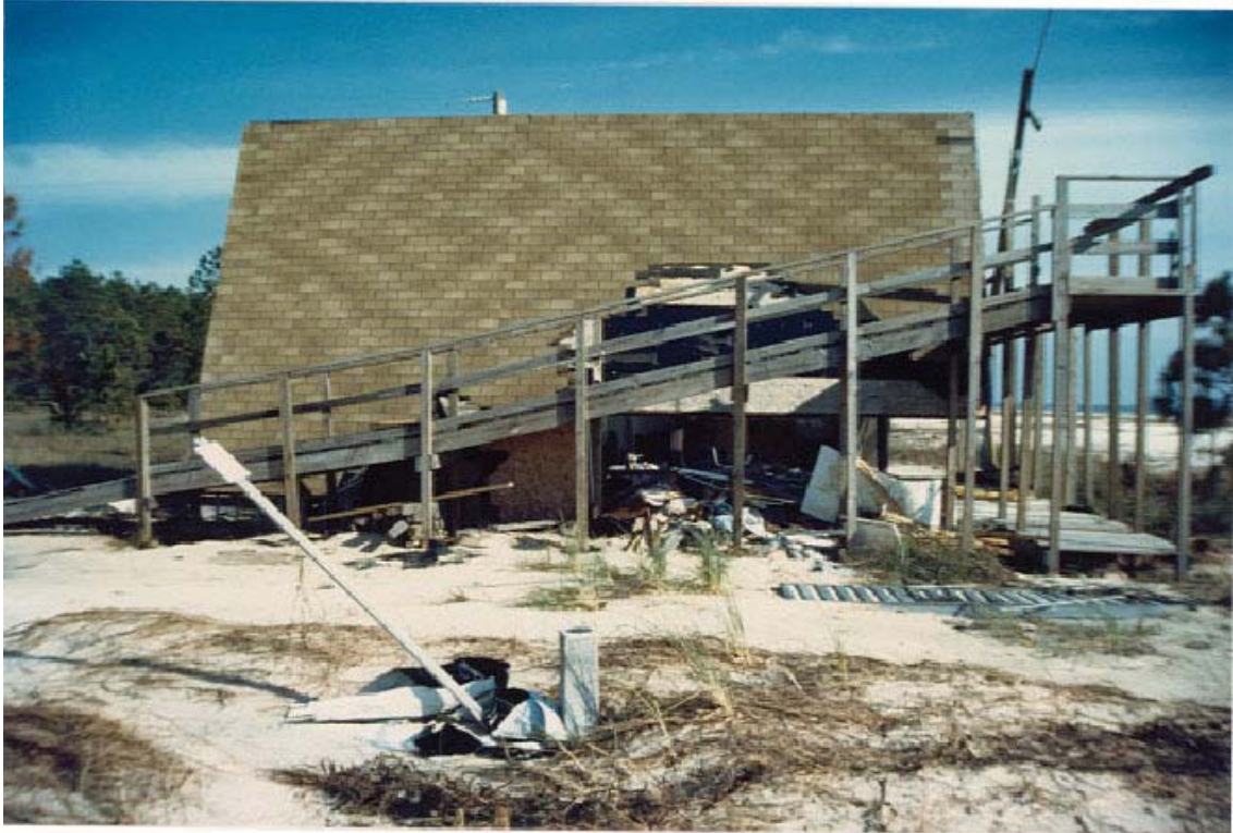
FIGURE 27. Dwelling damaged by wave impact loads.
