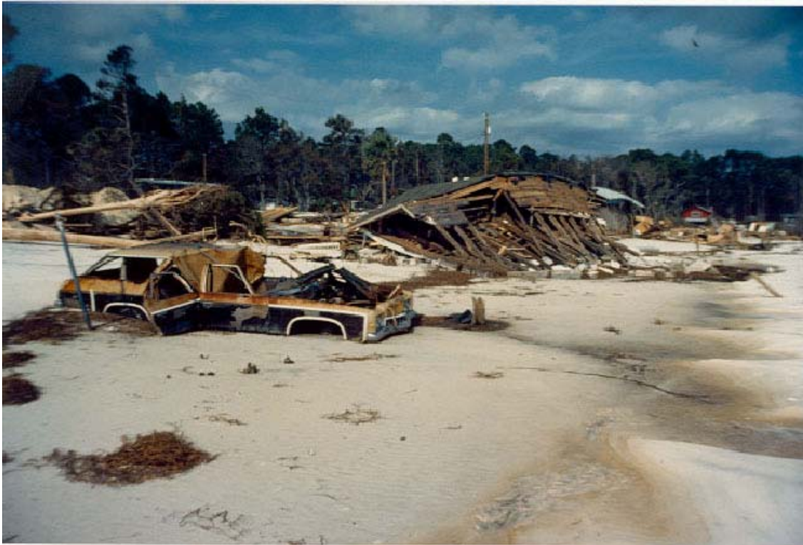
FIGURE 76. Severe damage west of Carrabelle Beach.
