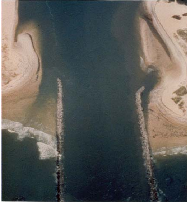
FIGURE 39. Sike's cut (St. George Island Channel) in November, 1985 prior to Kate (photograph by Kevin R. Bodge).
