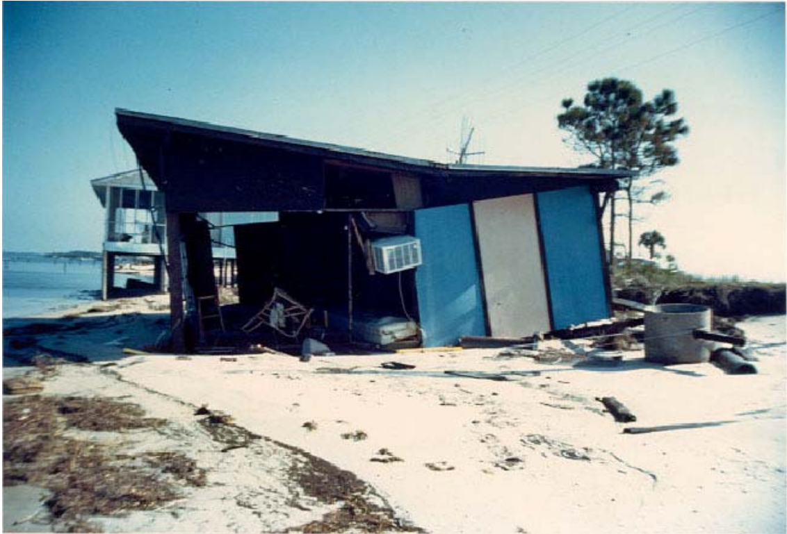
FIGURE 87. Alligator Harbor shoreline dwelling destroyed.
