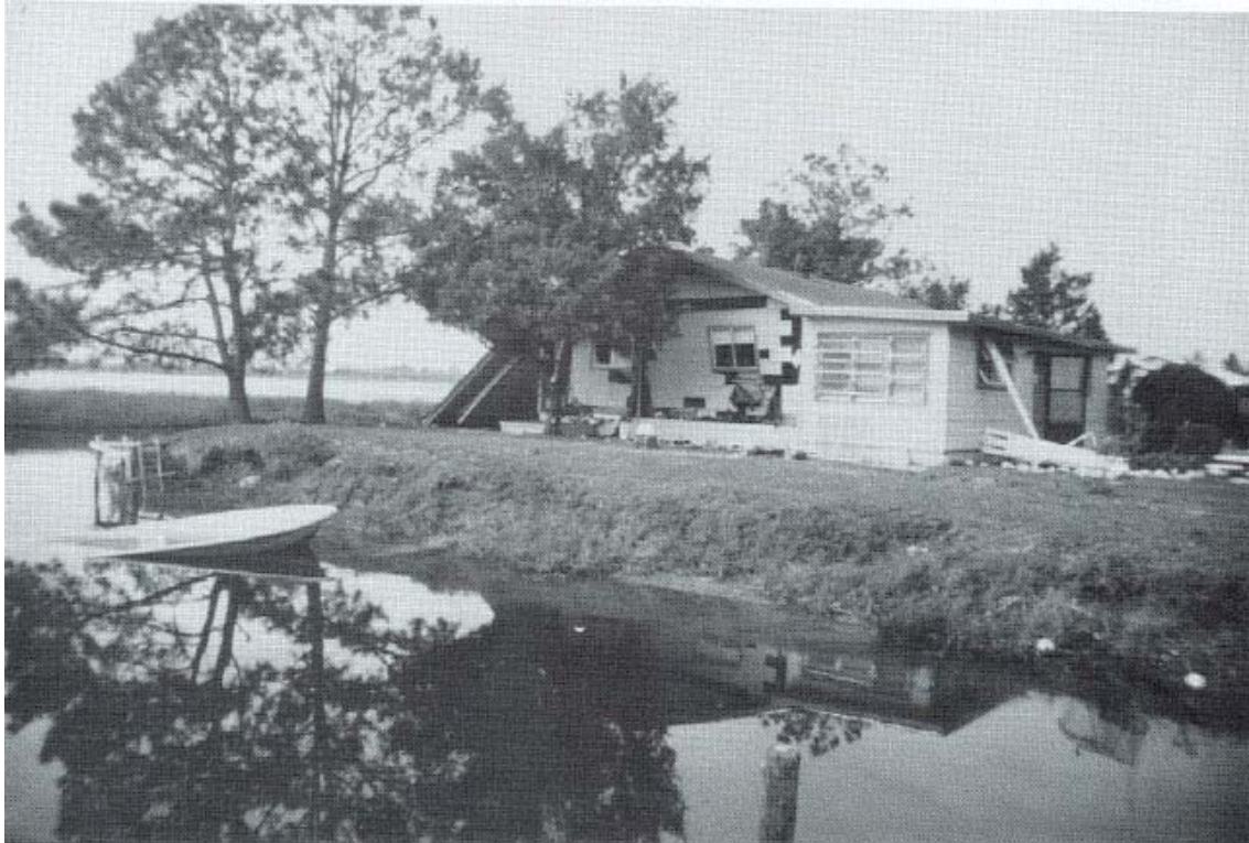
FIGURE 120. Dwelling damaged by waves which propagated across the island and the canal.
