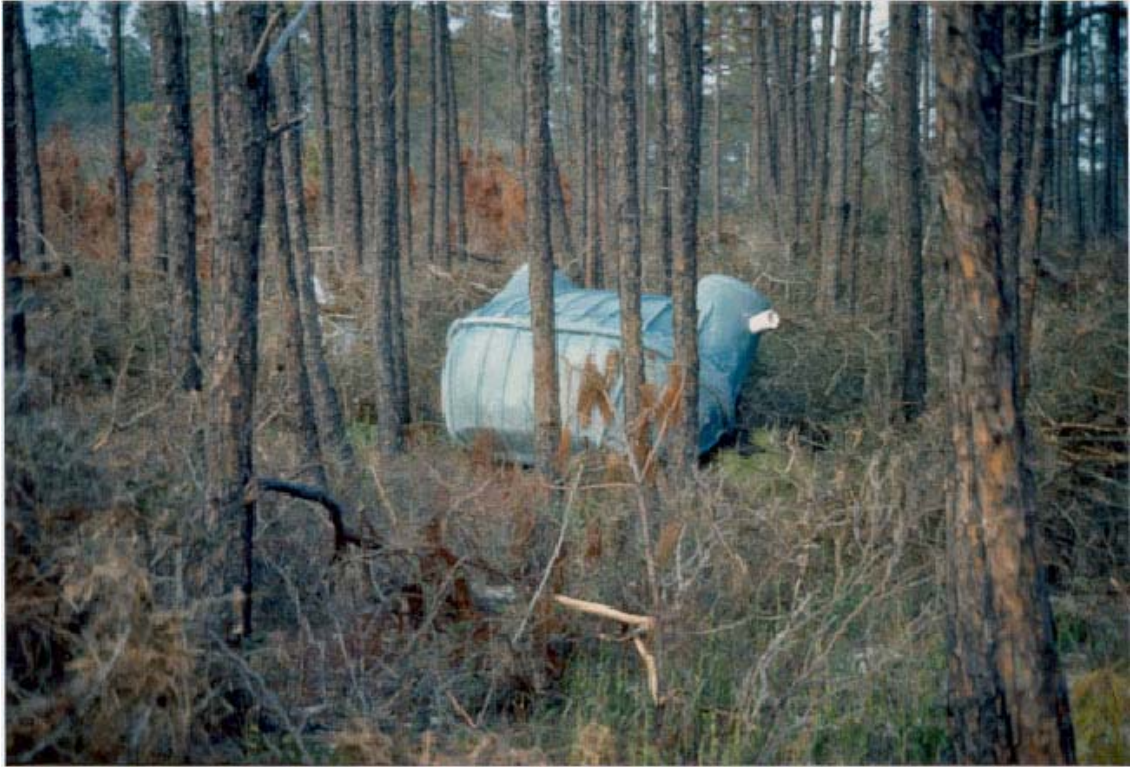
FIGURE 59. Dog Island septic tank carried inland by the flood.
